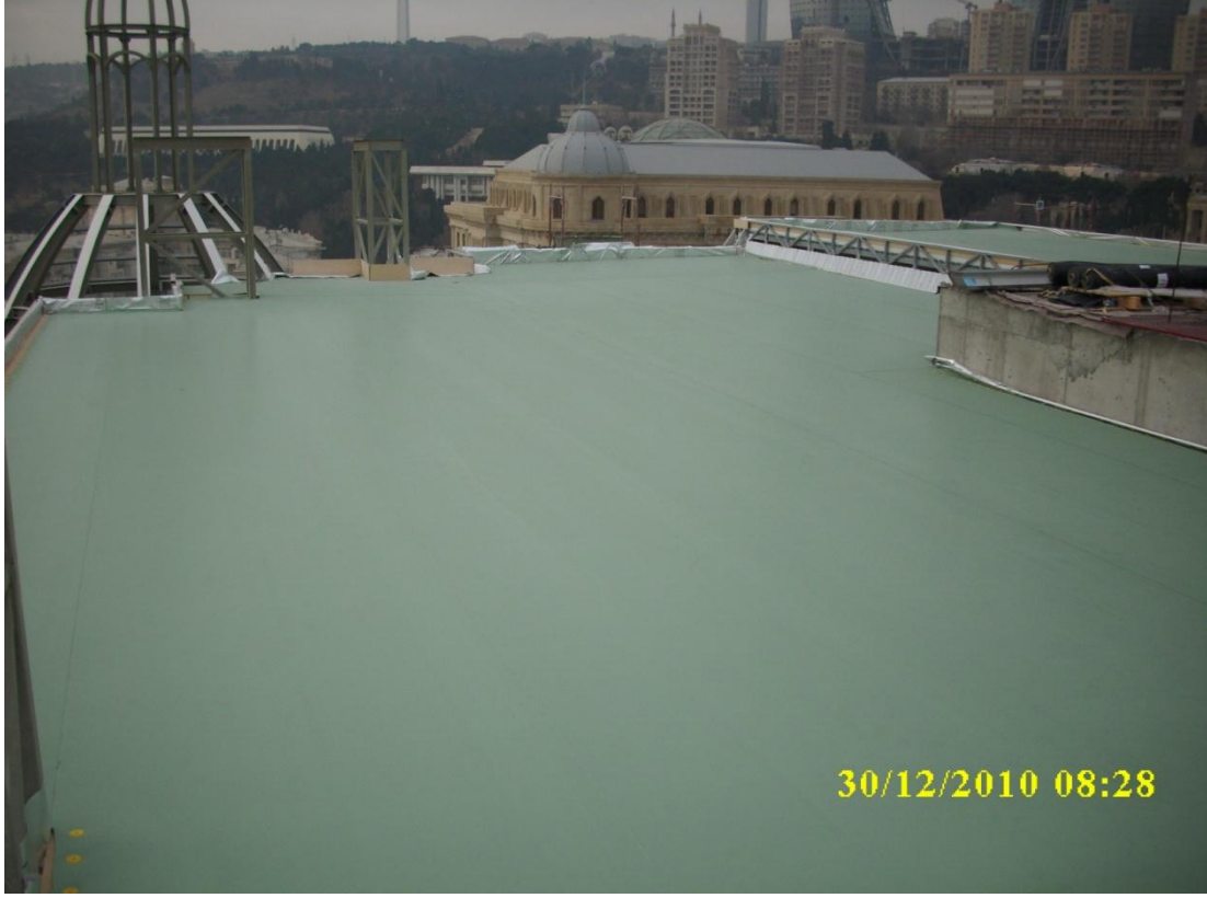
Application of PVC Single Ply Membrane
